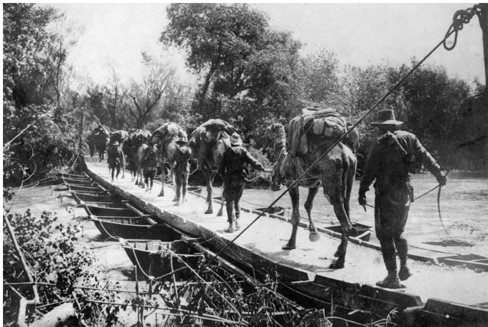
AWM P00190.004. Camel Corps crossing the River Jordan on pontoon bridge built by the Australian engineers.
